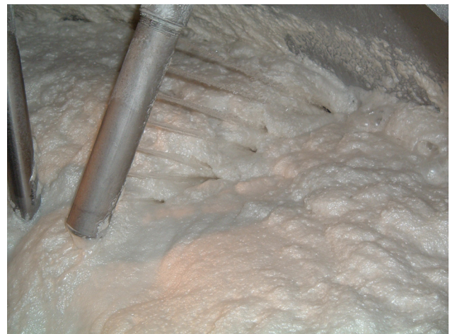
Figure 8: Froth washing installed on G-Cells
