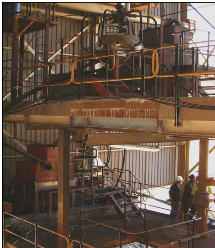
Figure 2: G-cell cleaner plant installation at Barbrook
